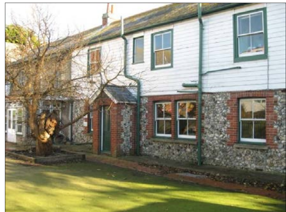
Curtilage listed terraced cottages
