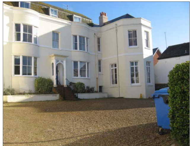
Small car parking area
